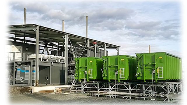
East Millinocket Biomass Power Generation
